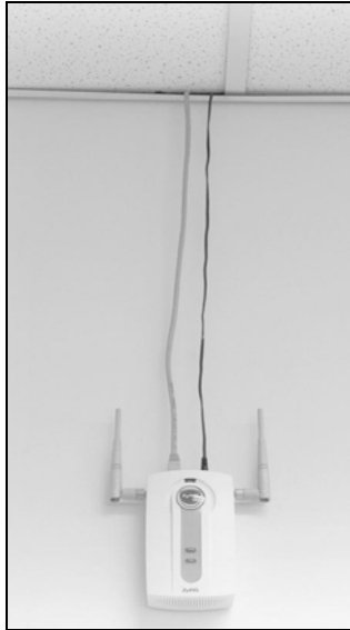
Figure 7 Run the Cables Upward
